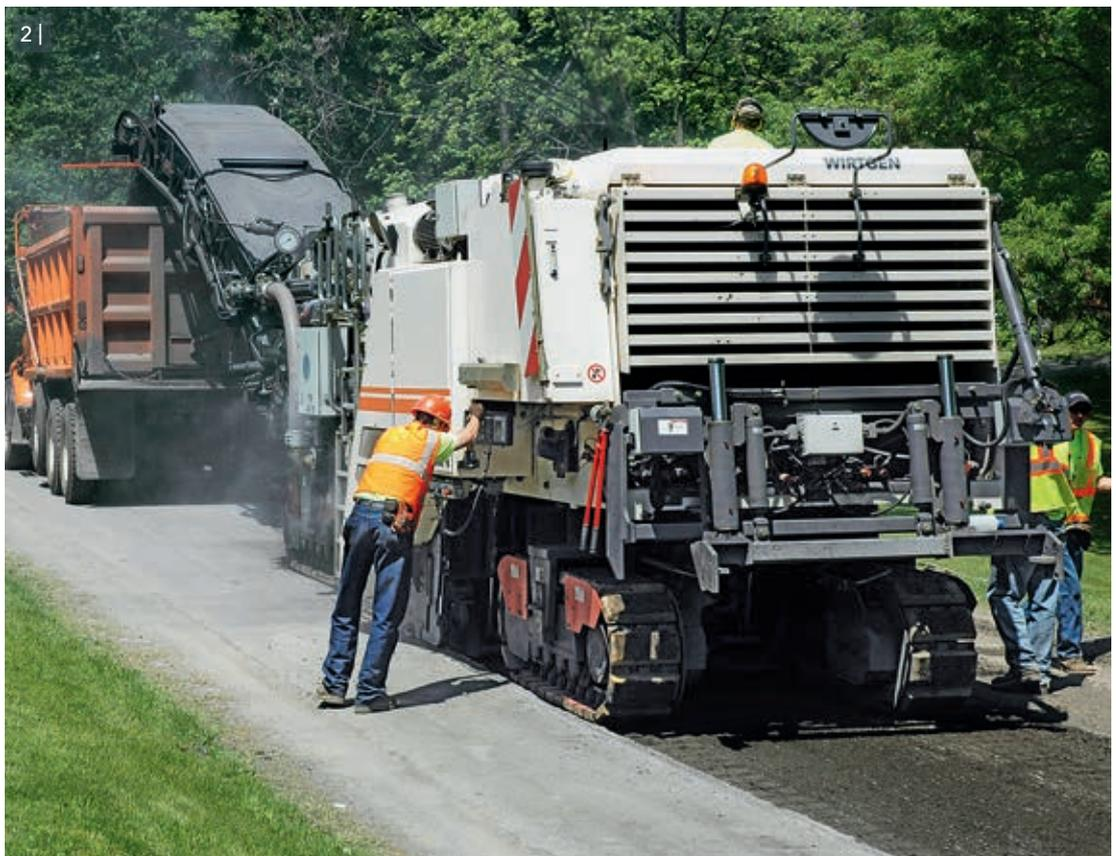
1 | As a high-performance in-situ cold recycler, the 2200 CR recycles asphalt roads in a single pass.
