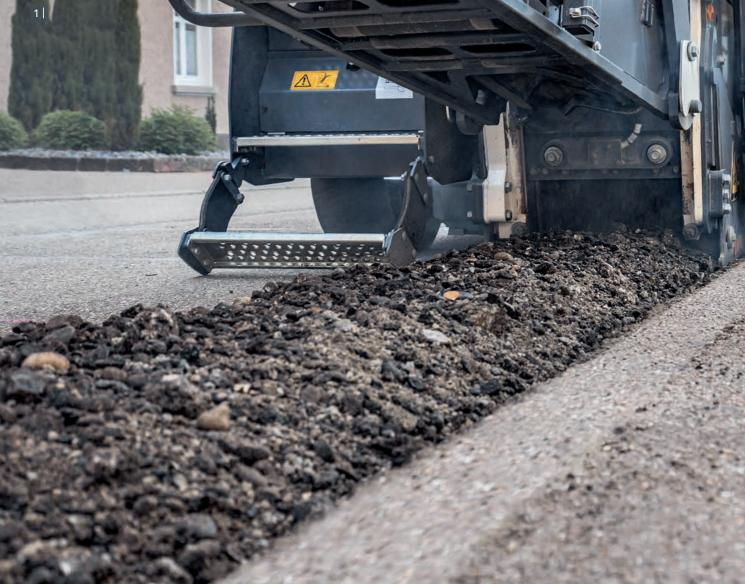
2 | Supplementary weights and tanks mounted in the centre of the machine ensure maximum traction in every job.
