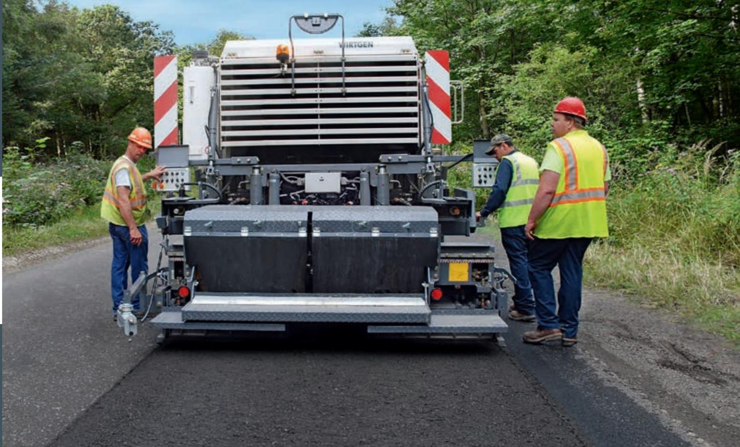
2.2-m wide paving unit with high-compaction VÖGELE paving screed and spreading auger.
