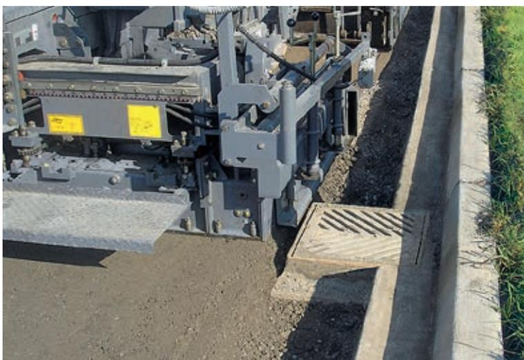
The centrally divided auger is operated in clockwise or counter-clockwise direction, the conveying speed of both sections being continuously adjustable. The screed's hydraulic tamper ensures reliable pre-compaction of the recycled pavement layer.
