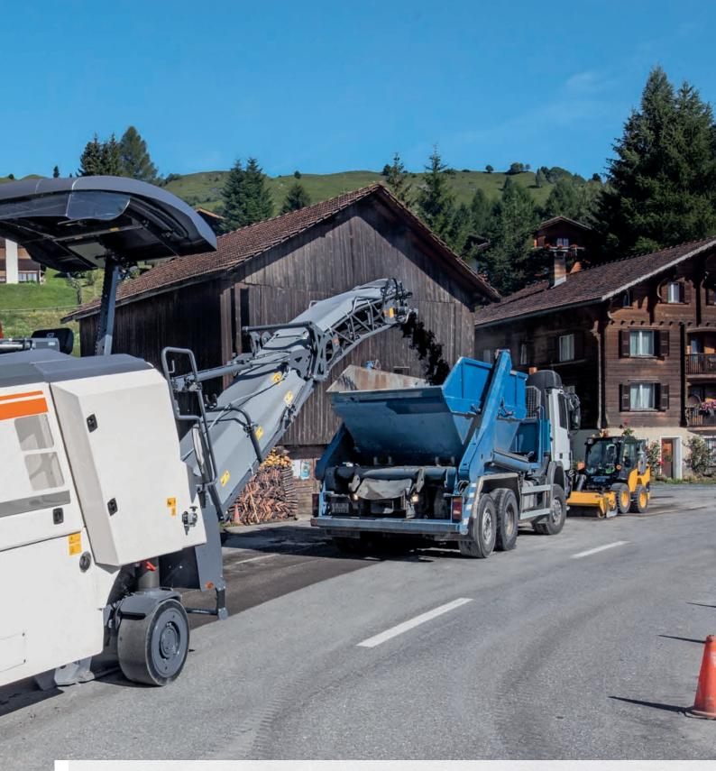
POWERFUL COLD MILLING MACHINE IN THE ONE-METRE CLASS FOR ECONOMICAL MILLING OPERATIONS AT A WORKING WIDTH OF 1.00 M OR 1.20 M.
