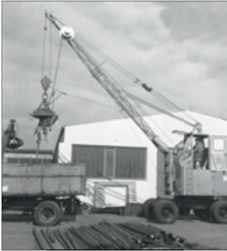
1962: rope-driven S833 with elevated operator cab
